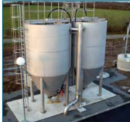
*The sand is returned by gravity to the top of the active sand bed after being routed downward through a labyrinth composed of several settling steps.*
