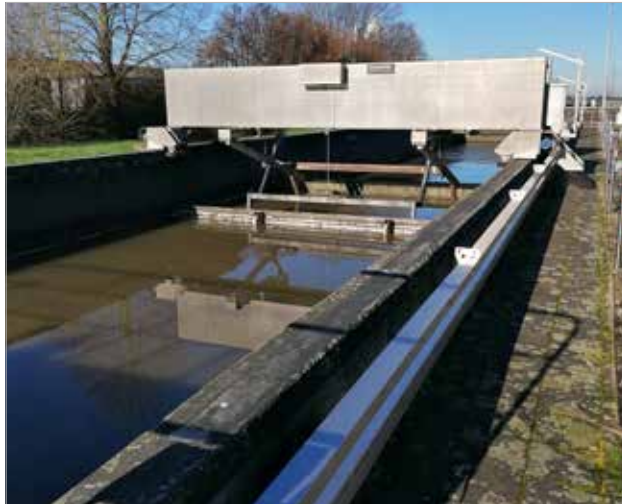
Räumerbrücke Scraper bridge
