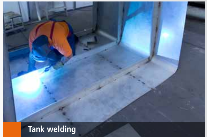
Welding on special equipment
