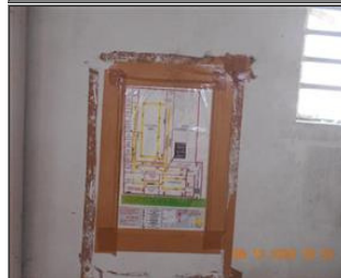
Photo of fire safety equipment DSCN4175.jpg
