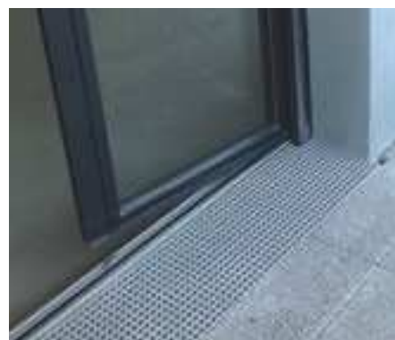
LOUVERED GRATING SHELVING, FENCING AND SAFETY RAILINGS
