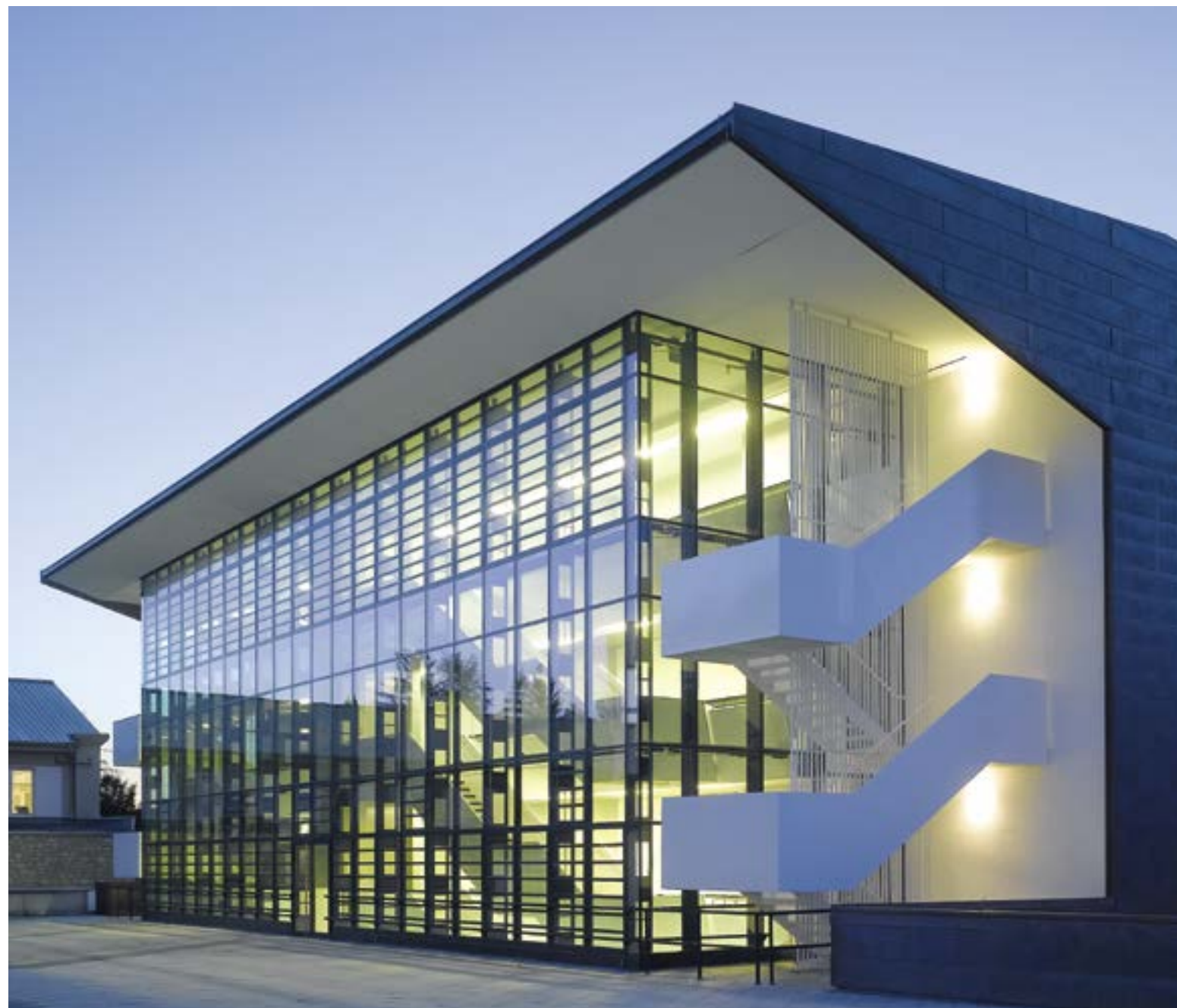
Deutschhaus School by Wulf Architects, Würzburg: The glazed stair hall allows the light to go as far as the ground floor. The louvre windows fitted in the façade provide dual-purpose day-to-day ventilation and emergency smoke release in the event of fire.
