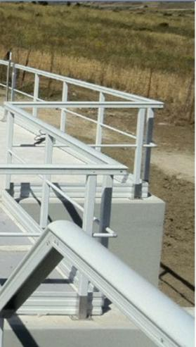
The handrail systems are made with pultruded profiles in isophthalic polyester resin and fibreglass.
