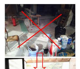
To provide an excellent impact protection (falling tools, scratch resistance, tire marks...) in a renovation building site with neither wrinkling nor easy tearing, just lay PP Diplast corrugated sheets (20sqm in 5 mn).
