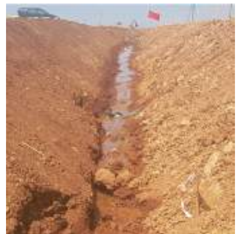
9. Drain pore water
