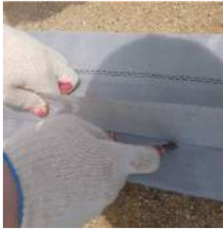
2. Form an insertion hole inside WHD wings
