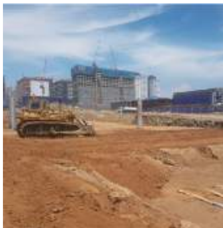
8. Place surcharge materials
