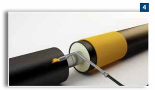
After welding, the outer surface of the casing is cleaned and heated with the torch.
